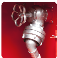
52 VALVE WITH SLANT REDUCTION
